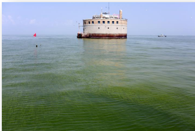
Toledo, OH water intake 2.5 miles from shore on Lake Erie (2014)
