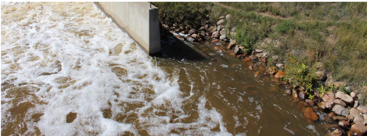
Figure 2 BCWA Site 45 Sampling Location below Weir.
