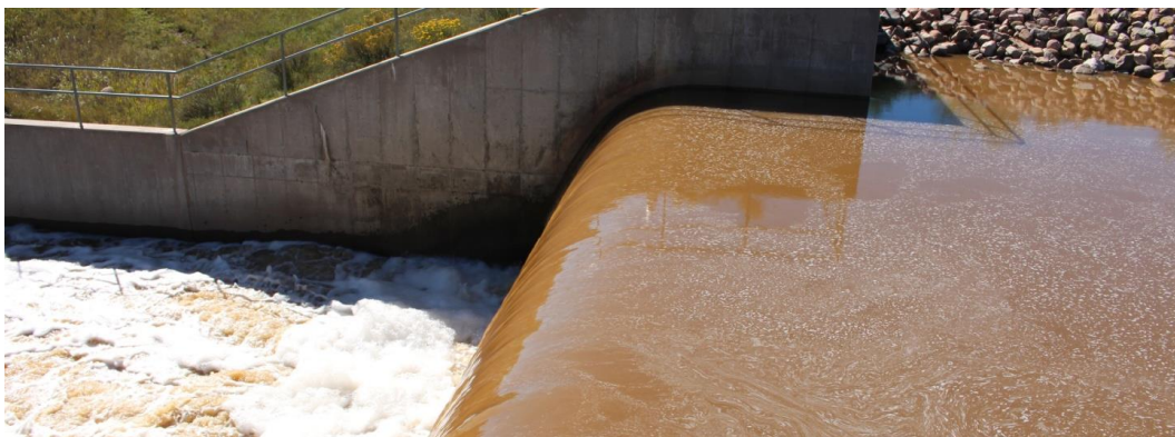
Figure 3 Heavy Sediment and Nutrient Load was Associated with 2015 Flows
