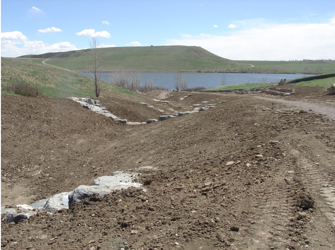
Figure 14 Coyote Gulch Construction Completion without vegetation
