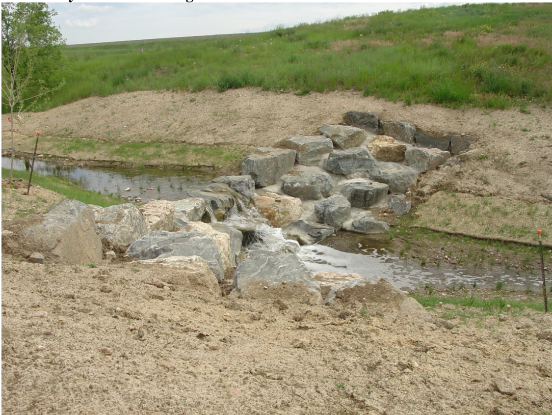
Figure 13 New Stone Check Dam Installed
