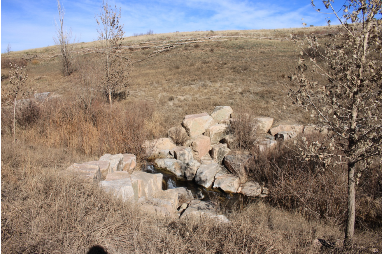
Figure 20 Rock drop structures not affected by submergence (November 2013)
