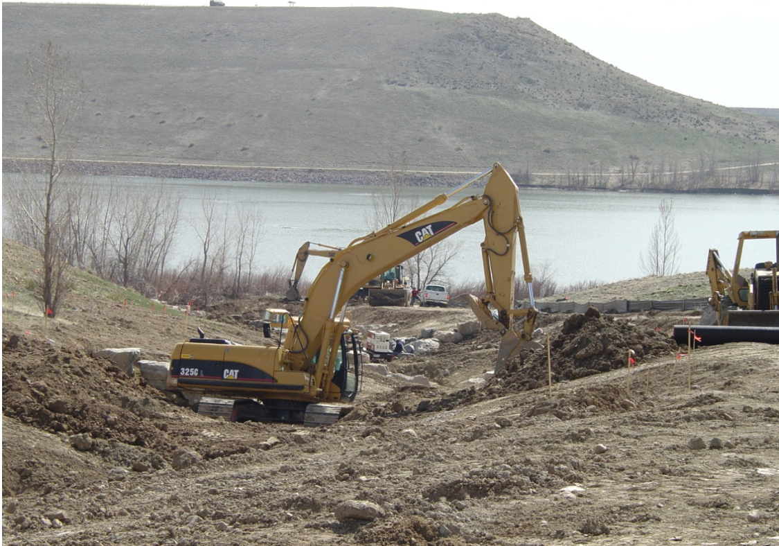
Figure 12 Coyote Gulch During Construction
