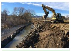
Lakewood completed stream bank restoration on Bear Creek caused by extremely high flows in 2015. By diverting flow around the project during construction, downstream water quality was protected.
