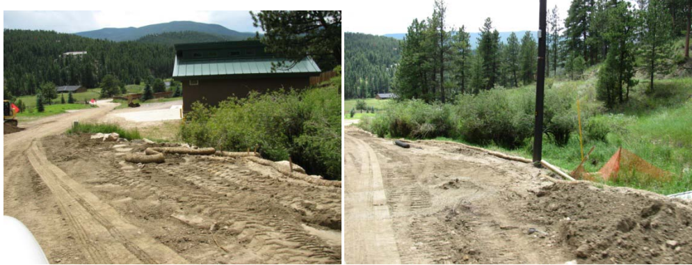
Figure 30 Potential Erosion and Drainage Control Problem in Clear Creek County
