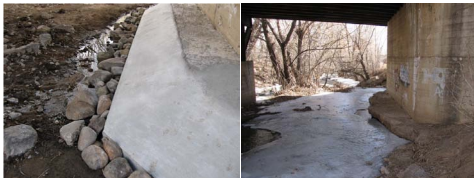
Figure 29 Runoff Controls Added To Bridge Repairs
