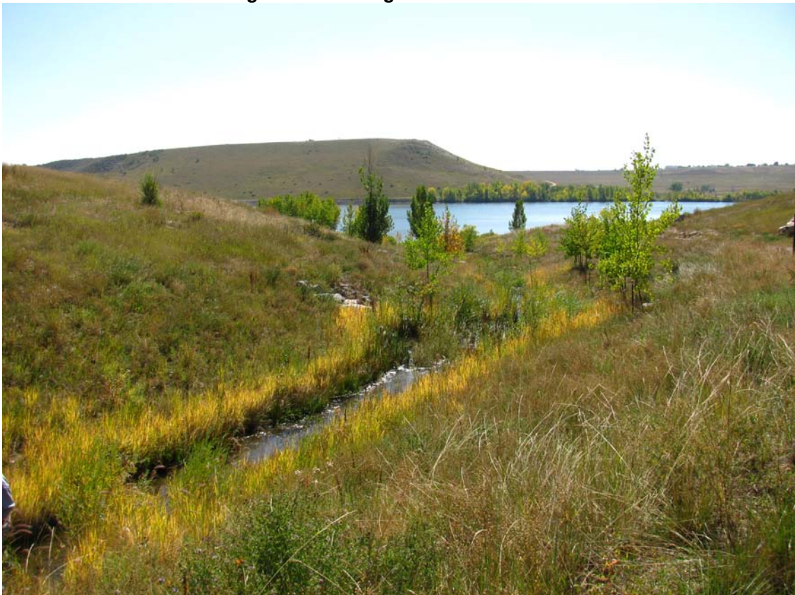
Figure 18 Coyote Gulch as Stabilized in Fall 2009
