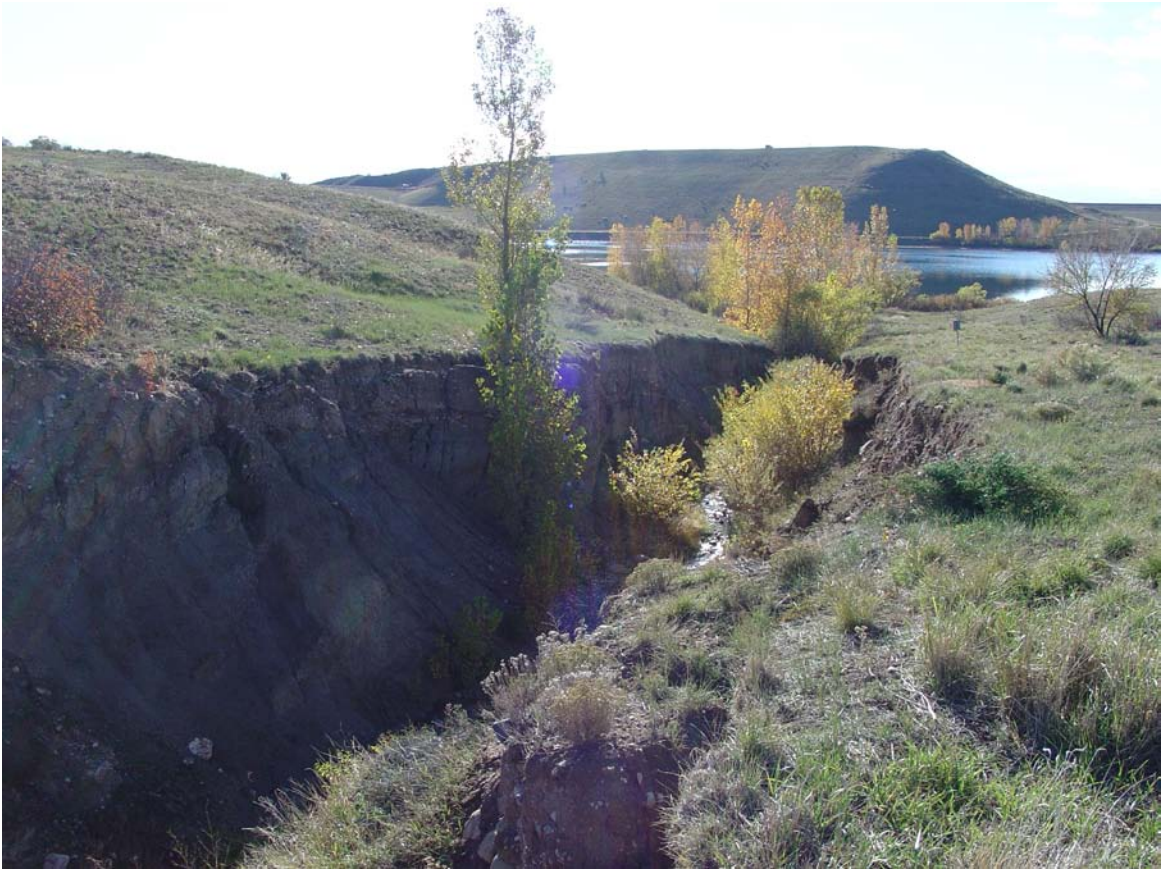
Figure 13 Coyote Gulch Pre-Construction
