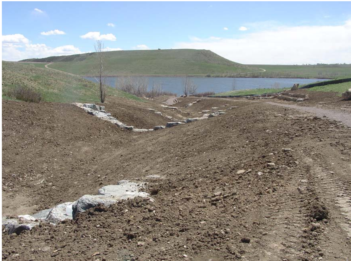
Figure 16 Coyote Gulch Construction Completion without vegetation
