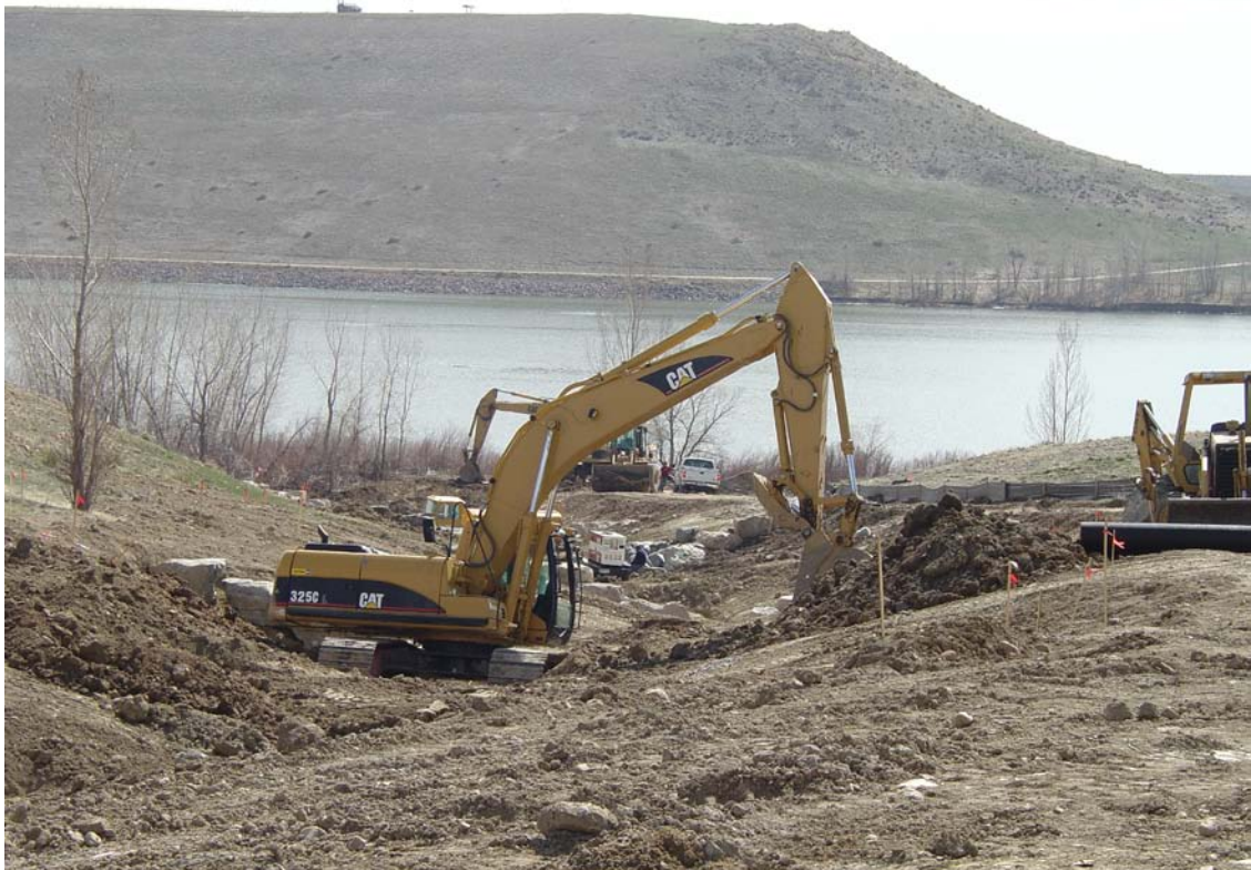
Figure 14 Coyote Gulch During Construction
