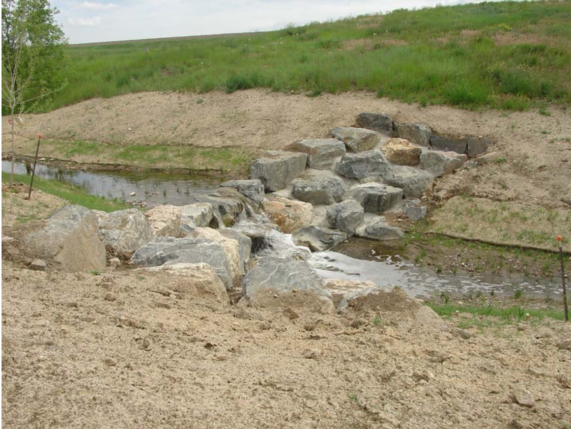
Figure 15 New Stone Check Dam Installed
